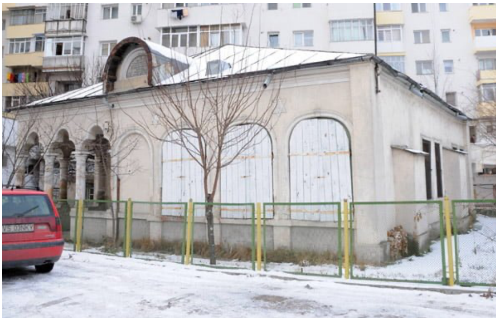
Vaslui Synagogue converted into a cultural center
